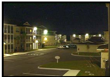
Parking Area from 2nd Floor
